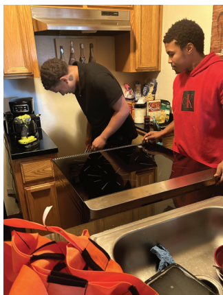
Range installation in progress
